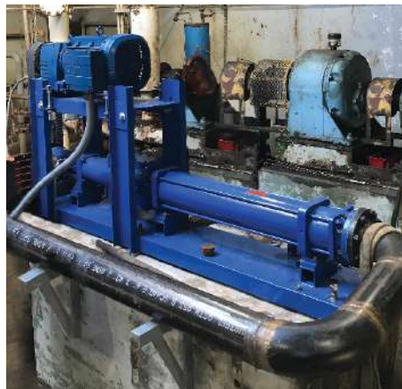
Above: MXQ EH Model Progressive Cavity Pump (Over & Under Package) installation
